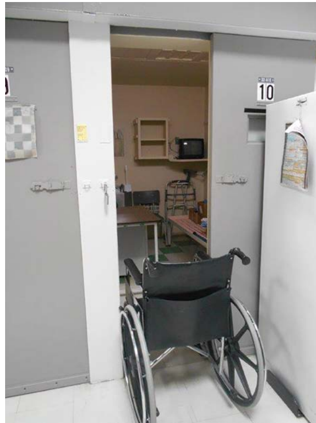
Wheelchair that cannot fit through a cell door – Federal Training Centre
